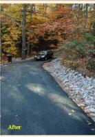
This high priority site experienced severe washouts with a direct flow to the lake. Installation of ditching on the west side of the road with new surface material and pavement mono-pitched towards the ditch. The Farley's also paved their severely eroding driveway which also contributed large amounts of sediment to the lake.
